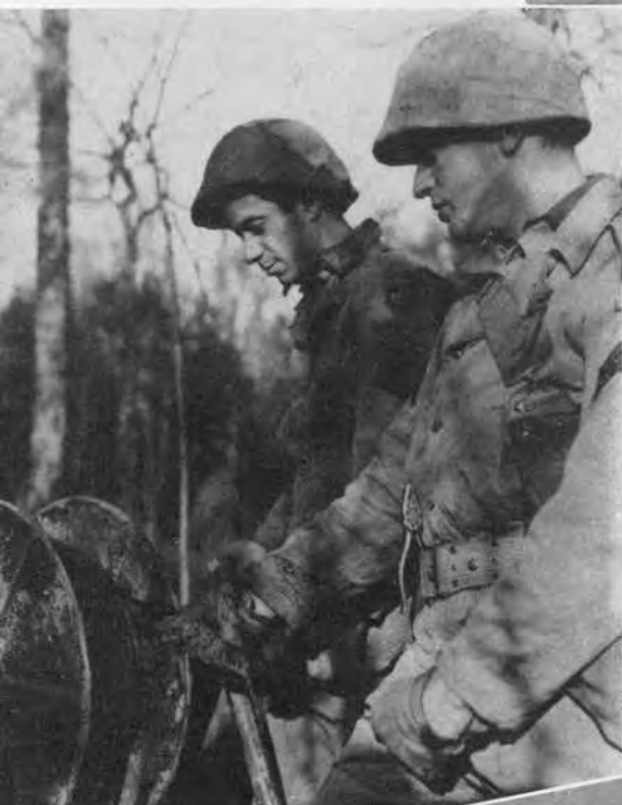
T and T servicing wire.
