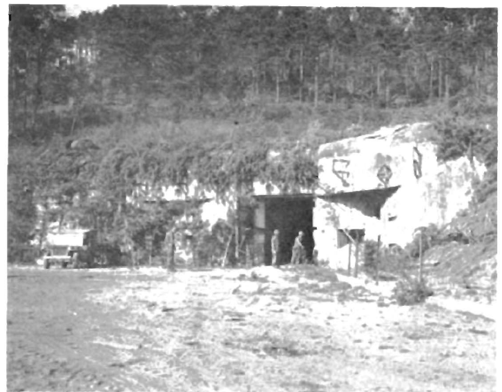
Closeup of entrance to mammoth Ft. Osterbeil. Note thick walls and ingenious construction into side of hill affording minimum target.
